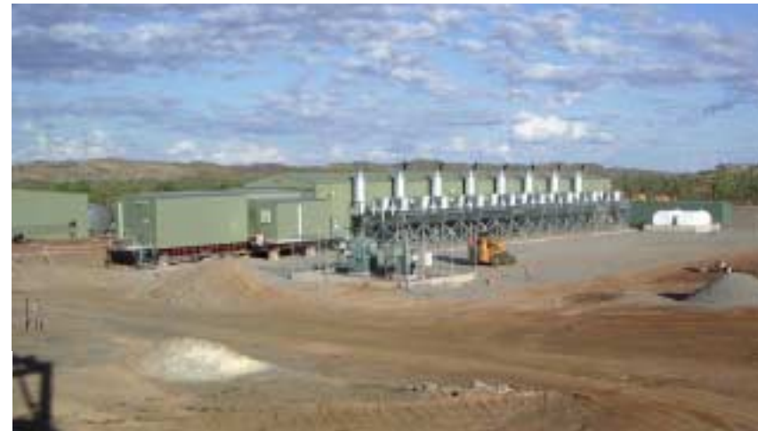
Above: Overall view of Sally Malay power station with control and switch room at left hand side.
