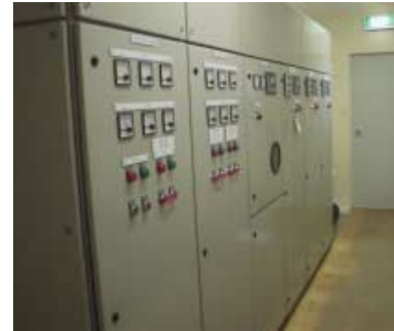
Above right: An early power station control panel, which contains three IntelliGen controllers only
