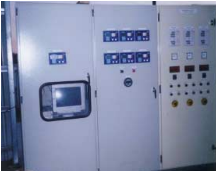
Above right: An early power station control panel, which contains three IntelliGen controllers only
