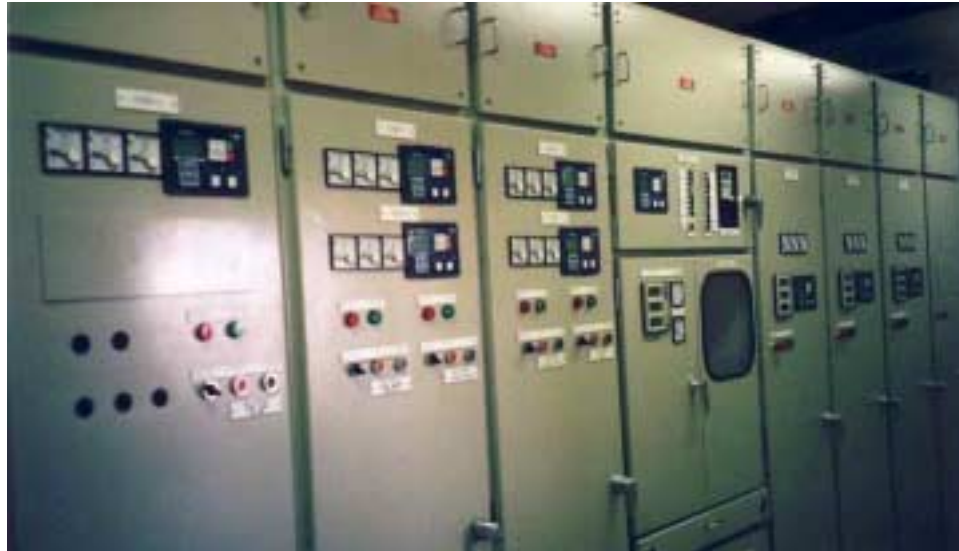
Left: A major new switchboard comprising three IntelliGen genset controllers (with space for a fourth), five Feeder Control Units and a Power Station Controller plus a PC running Winedit/MultiEdit and IG-LOG logging program.
