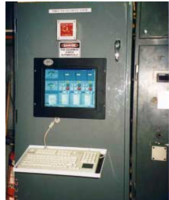
Left: A major new switchboard comprising three IntelliGen genset controllers (with space for a fourth), five Feeder Control Units and a Power Station Controller plus a PC running Winedit/MultiEdit and IG-LOG logging program.
